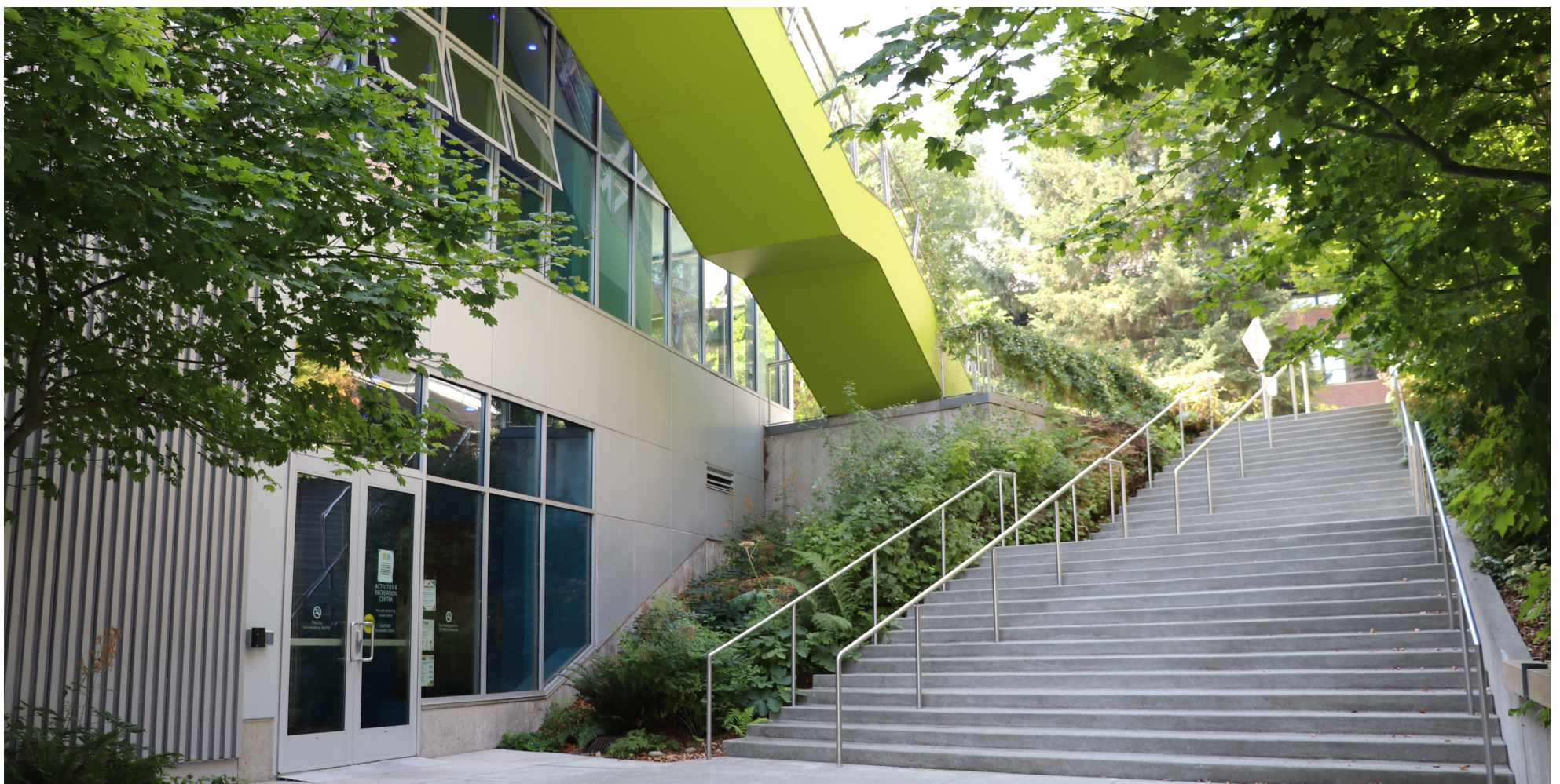
Entrance to the Lower Level of the ARC
